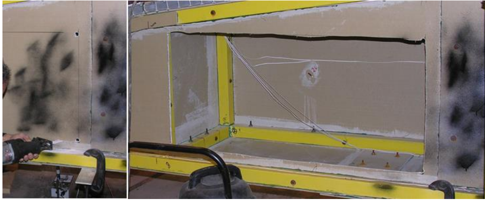
Figure 4-16: Bridge Damage created using a reciprocating saw
