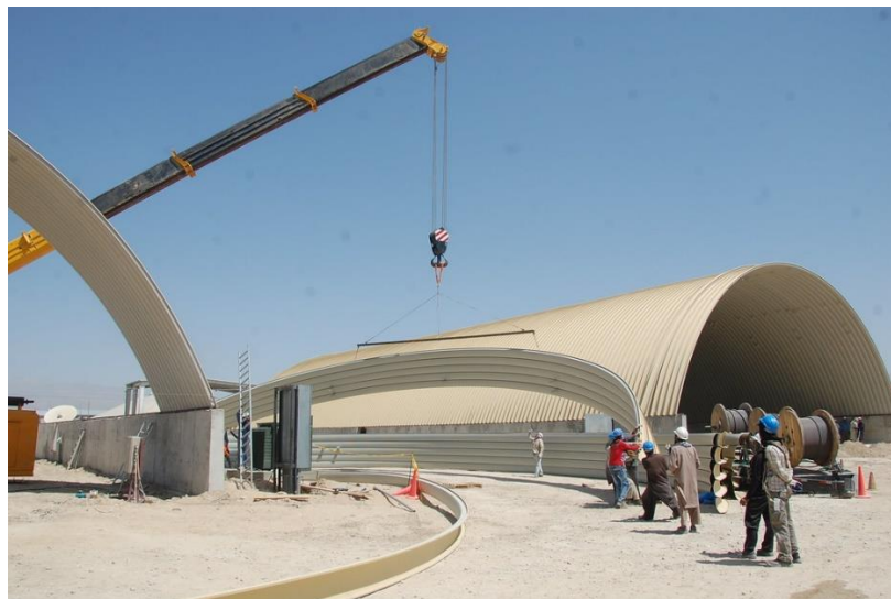
Figure 2-3: Erection Process of K-Span [8]
