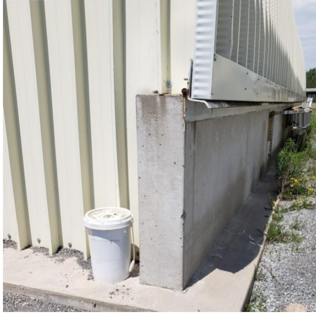
Figure 2-15: CFB Kingston K-Span Steel Hinge Support Connection
