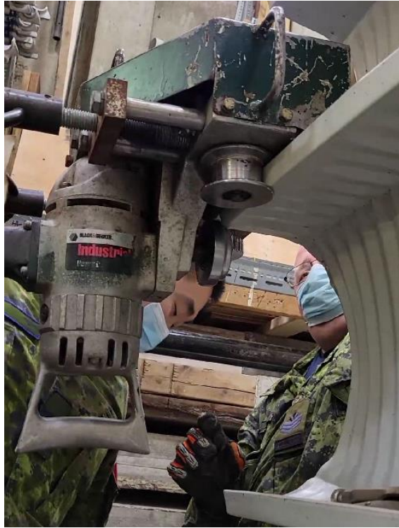
Figure C-7: Beginning of Seaming Process
