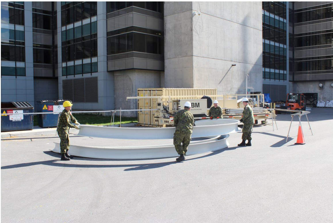
Figure C-4: Scale of 7m-Diameter Panels on Jobsite
