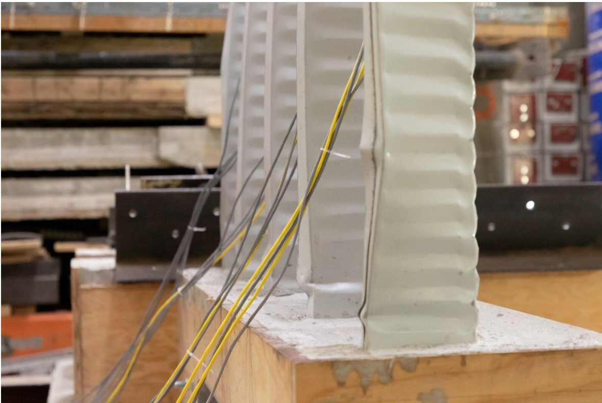
Figure C-28: Balanced Loading & Fixed Support Specimen Localized Buckling near Supports
