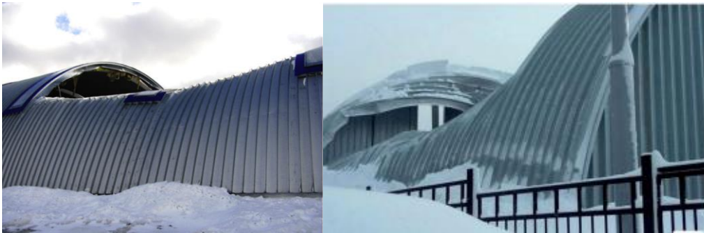
Figure 2-11: K-Span Collapse Gdansk, Poland [14] (Left) and Yuzhno-Sakhalinsk, Russia [15] (Right)
