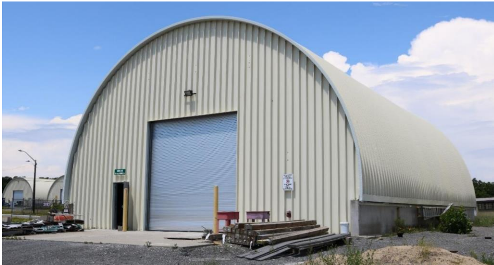
Figure 4-1: K-Span Structure (Photographed by G. Lépine [16])
