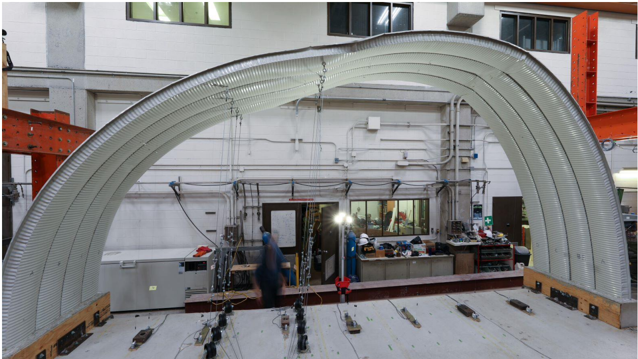
Figure C-40: Unbalanced Loading & Fixed Support Specimen During Loading
