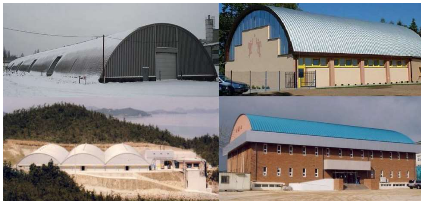
Figure 2.1 - Various civilian usage of K-Span structures [8]
