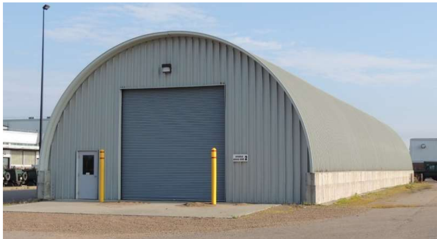
Figure 1.1 - K-Span structure in CFB Petawawa [2]
