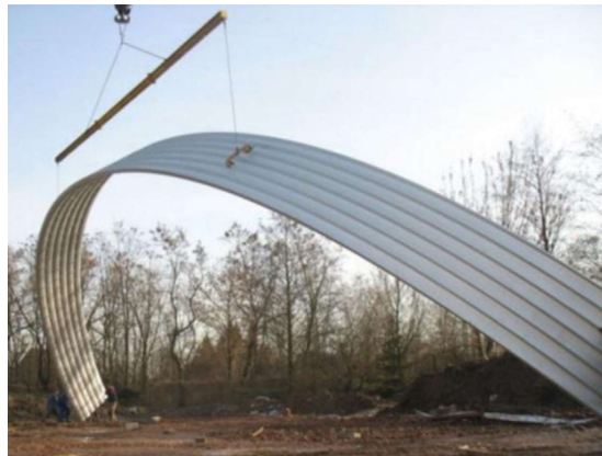
Figure 2.9 - A set of six seamed MIC-120 panels erected by crane [8] [15]
