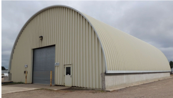
Figure 3.1 - Example of MIC-120 K-Span structure at CFB Petawawa [4]
