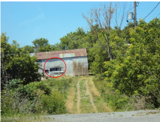
12 viewed from south
