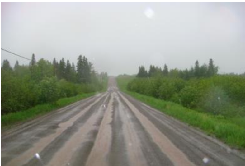
Image 9 (Left). Main road in Kerr Brook during rainfall event. Slightly rutted with long slope length.
