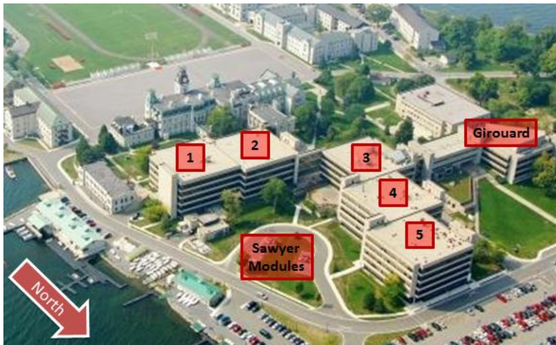
Figure 1.1 – Sawyer and Girouard buildings prior renovations (Structural tender drawings, 2010)
