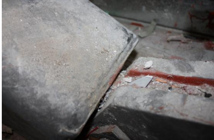
Figure 4.27 – Lower connection installed
