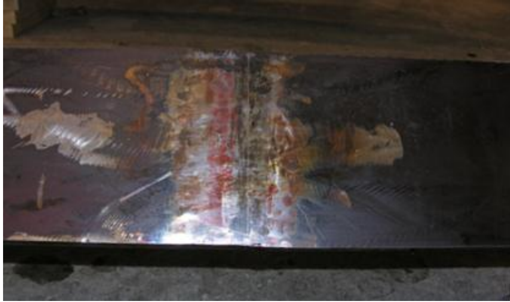
Figure 3.11 – BR6 weld at mid-span
