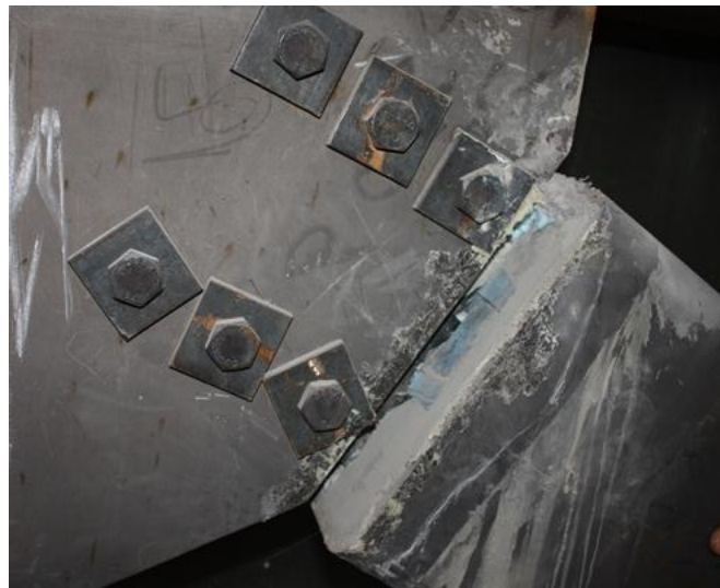
Figure 4.26 – Upper connection installed
