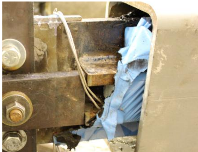
Figure 3.31 – Un-bonding membrane adhesive failure
