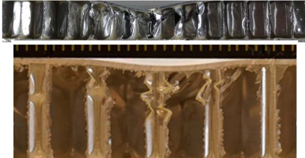
Figure 1-2: Surface denting and core damage due to impact [2, 3].
