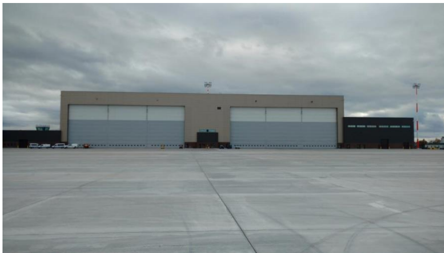
Figure B.5: Hangar 6 (B606)
