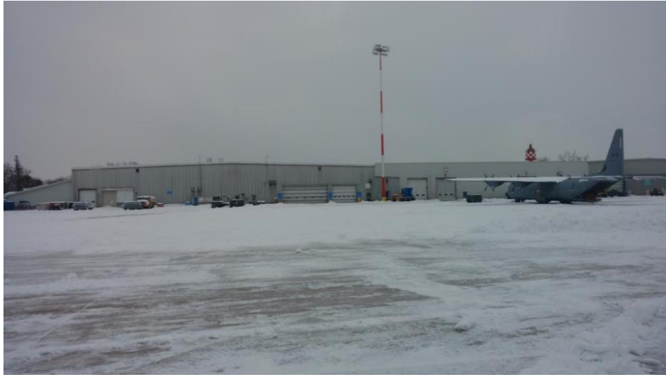
Figure B.11: 2 Air Mov Sqn Freight Reception Centre (B066)
