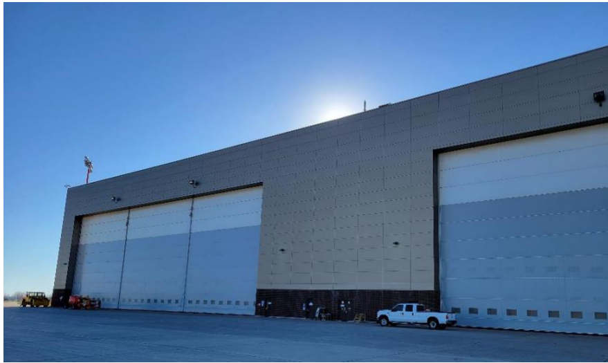
Figure B.4: Hangar 2 (B607)
