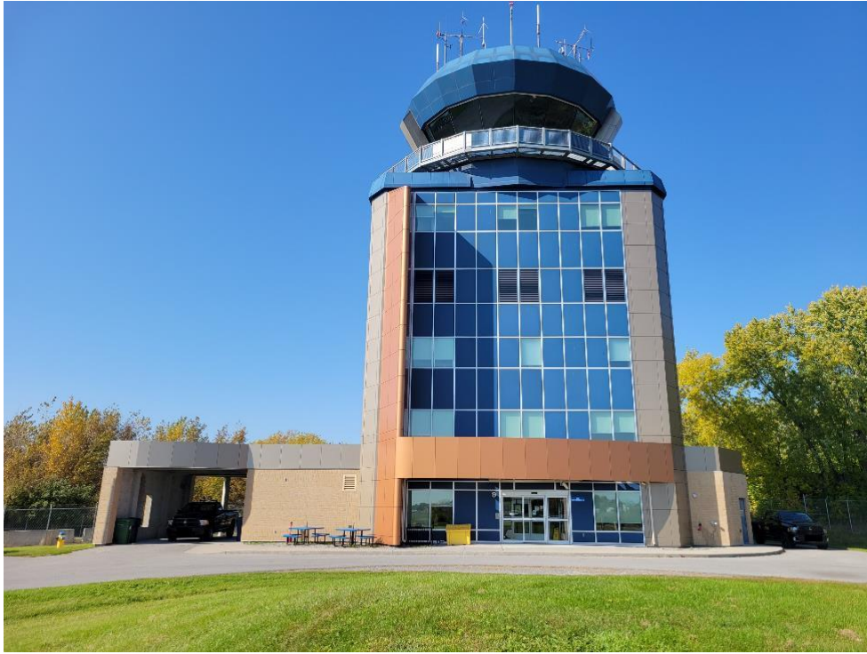
Figure B.15: 8 OSS, Control Tower (B478)
