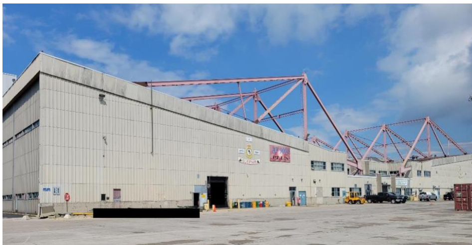
Figure B.9: Hangar 10 (B052)
