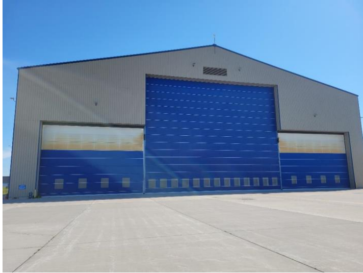
Figure B.2: Hangar 7, CC-177 Interim Maintenance Hangar (B522)
