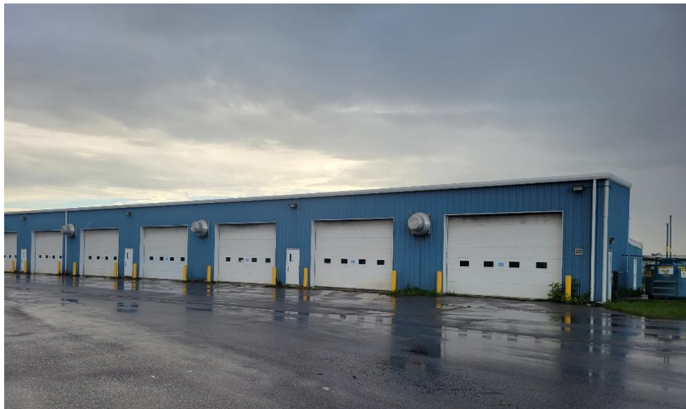
Figure B.14: Refuelling Depot (B354)
