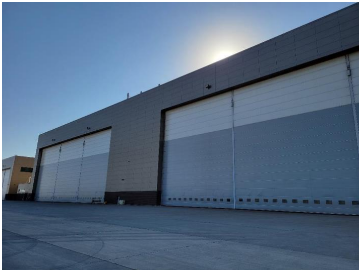
Figure B.3: Hangar 1 (B575)
