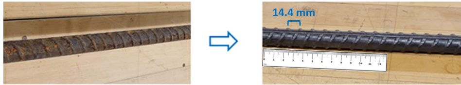
Figure 4-4. Rebar cleaned of rust
