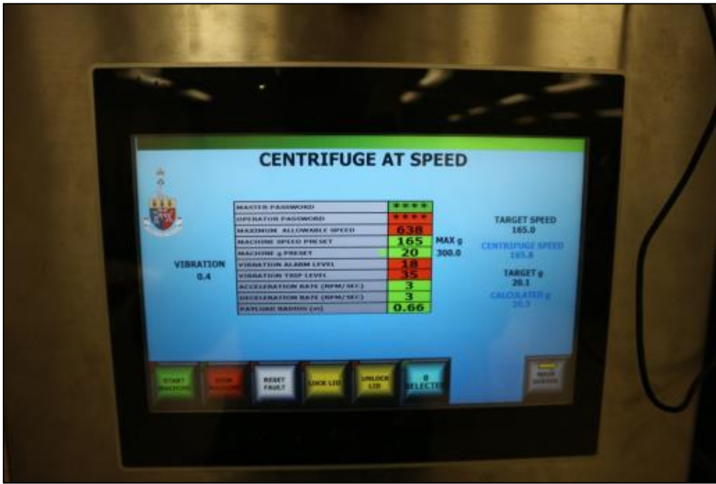
Figure D-86: Centrifuge at speed.
