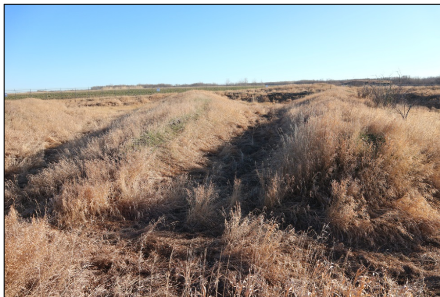
Figure 4.12- Site condition of derelict sludge drying beds
