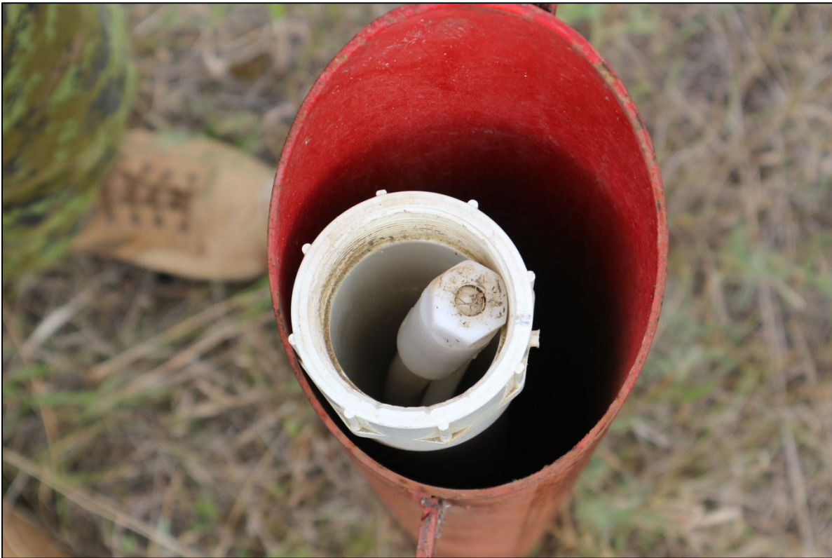
Figure F11 – Example of a Waterra pump and tubing found within some of the MWs (SL#1).
