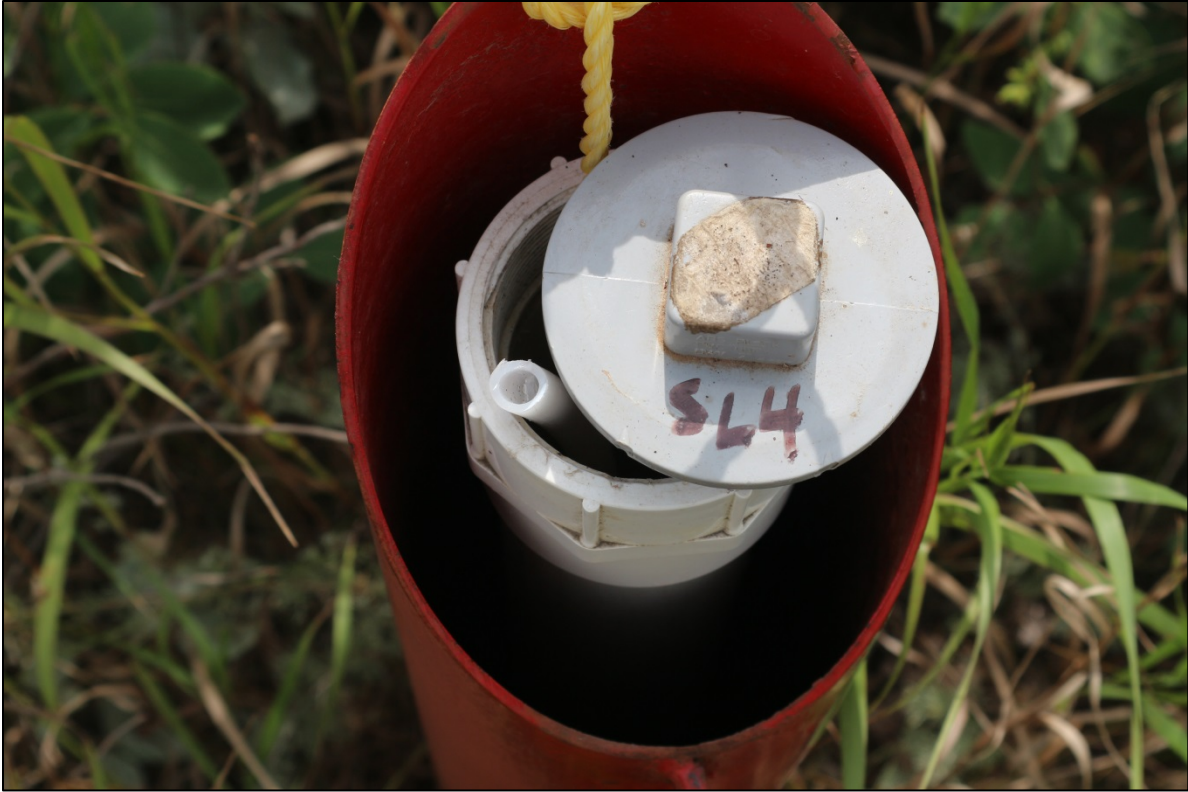
Figure F12 - Example of sampling equipment found preventing the lid of the MWs to be properly secured (SL#4).
