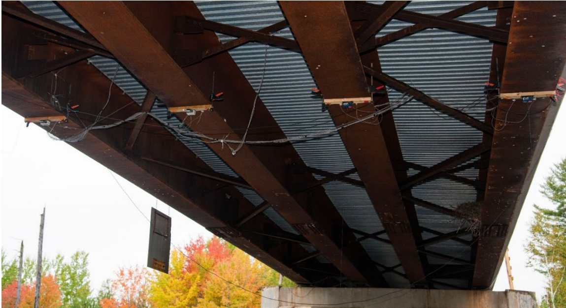
Figure A - 12. View of L3 Instrumentation from East Abutment.
