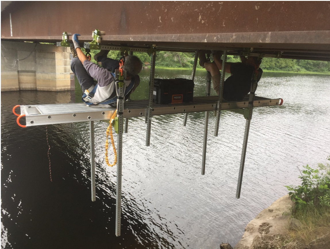
Figure B - 2. Platform in-use on Bridge.
