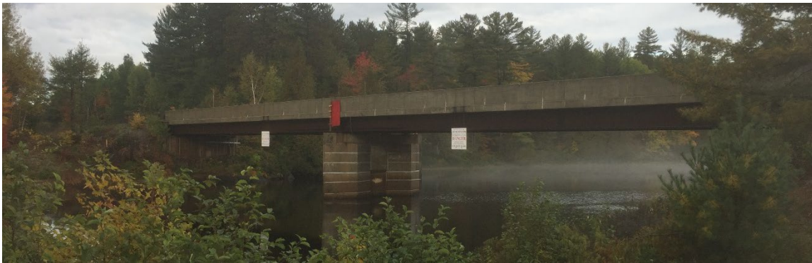
Figure 4-6. Elevation View of the Mountbatten Bridge from the South-East Shore.
