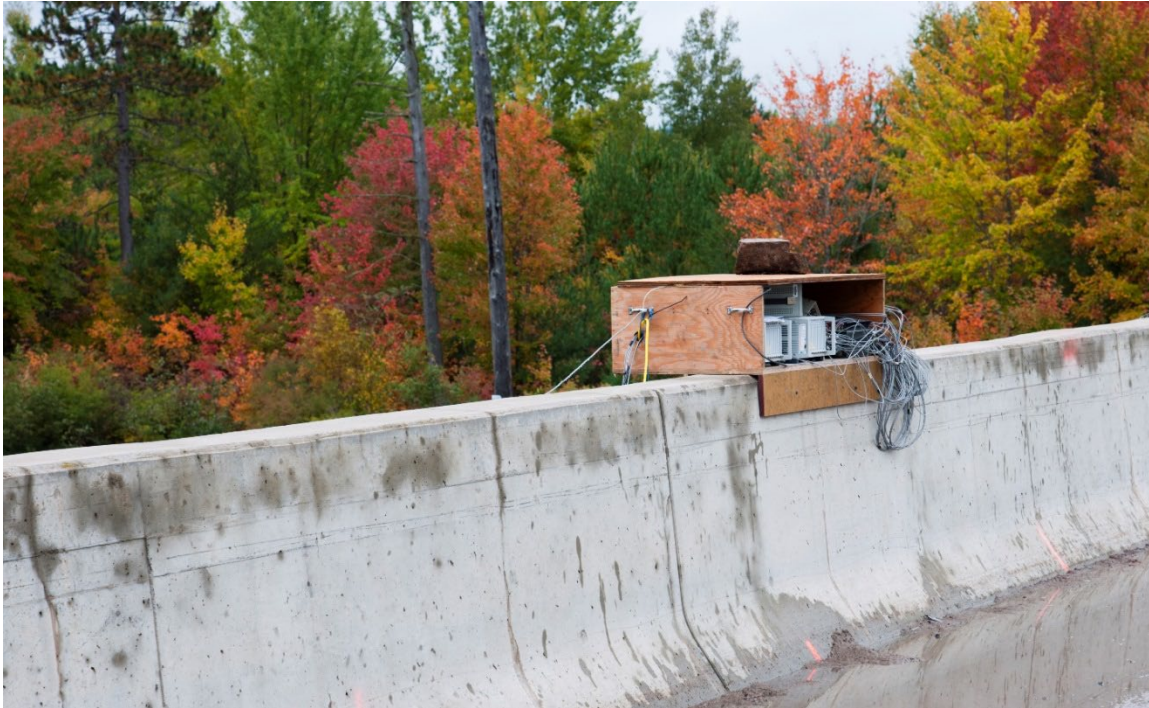
Figure A - 14. DAQ at L3 from Bridge Surface.
