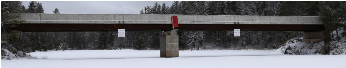
Figure 3-7. Elevation View of the Mountbatten Bridge in Winter.
