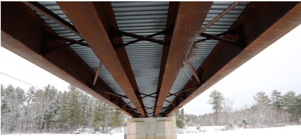
Figure 3-10. Underside of the Mountbatten Bridge from East Abutment.
