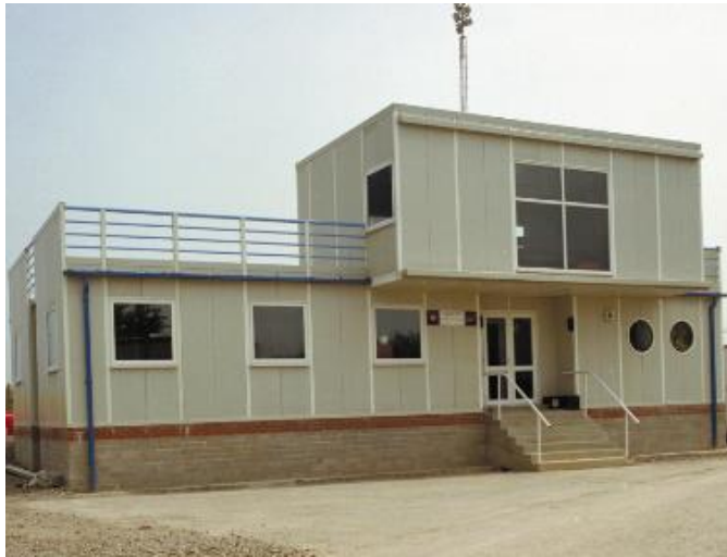
Figure 3.1 - A visitor center in Bristol, UK constructed with COMPOSOLITE® panels [4]
