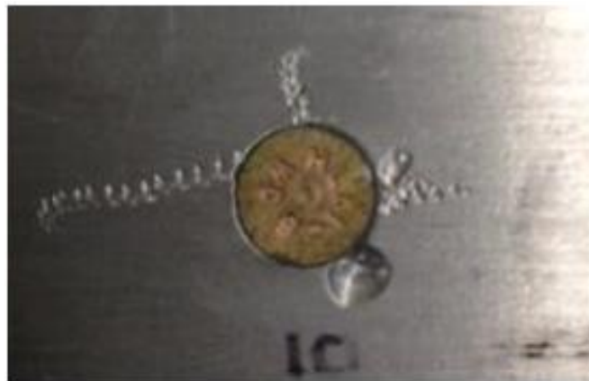
Figure 2: Example of typical damage that may be incurred by drill bit on aluminum surface of lap-joint structure during ferrous fastener removal process [10].
