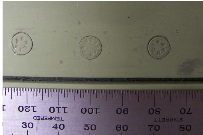
Figure 54: Visible fastener damage encountered on NAVAIR sample.
